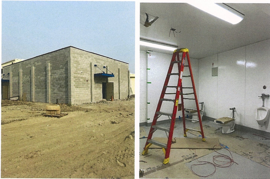
Exterior View of Girls Side and New Restroom Area Boys Side
